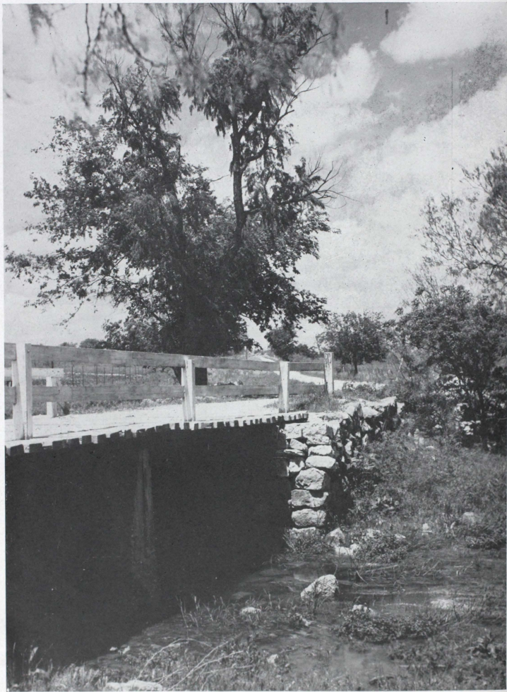
Across the Bridge to the Maneuver Area
