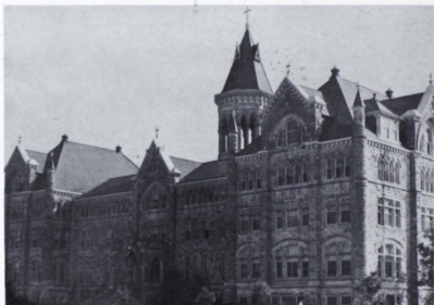
Main Building: The Stone Giant.
