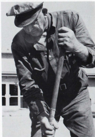
Oscar Krull and another broken water main.
